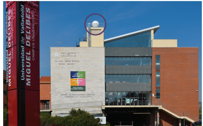
Dartcom X-Band EOS System at the University of Valladolid, Spain, with antenna (circled) installed on a lift shaft
