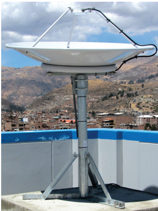
Dartcom 1.25m parabolic dish antenna installed at the University of Huaraz in Peru
