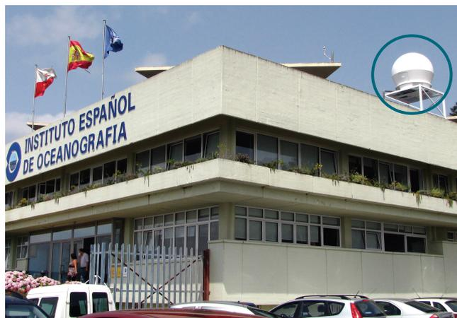
Dartcom HRPT/AHRPT System at the Spanish Institute of Oceanography, with a radome-enclosed 1.5m antenna installed on a roof-mounted platform (circled)
